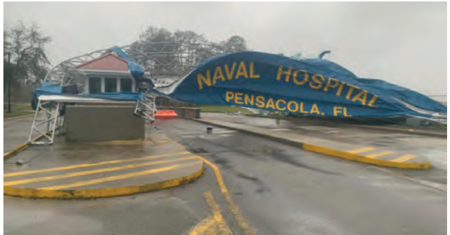
Naval Air Station Pensacola sustained water and wind damage from category 2 Hurricane Sally. The storm landed in Gulf Shores, Alabama on September 17, 2020. Photo by Naval Hospital, Pensacola
